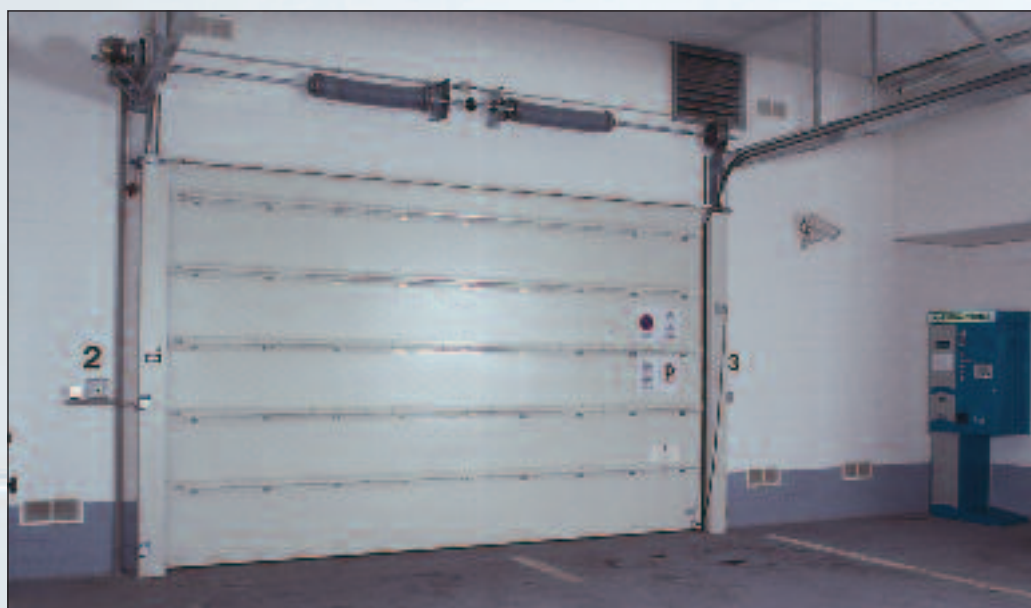
T30 Sectionaltor in Tiefgarage.
